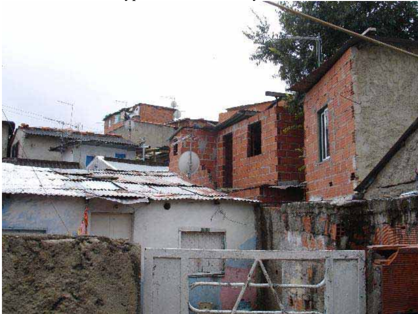
As time pass by more floors are added to the initial houses
